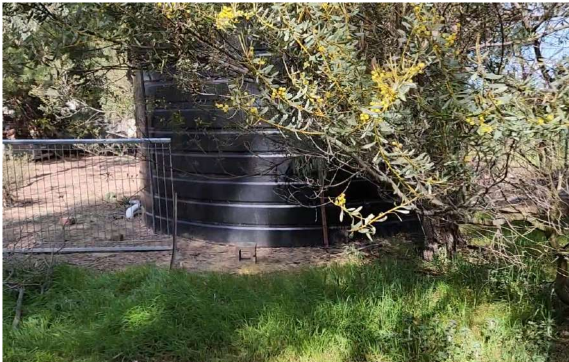
Photo 5 Existing holding tank with a capacity of ~43,320L.
